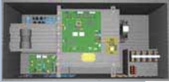
Set Free units electrical control box
