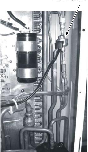
Electronic expansion valve coil
