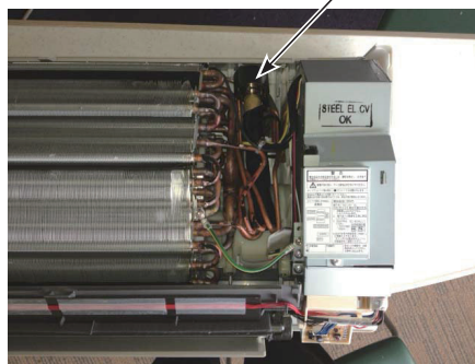
Electronic Expansion Valve Coil
