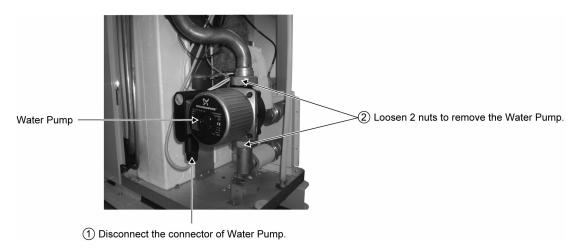
⚠ When reinstall the water pipe, use grease or water at the joining.
